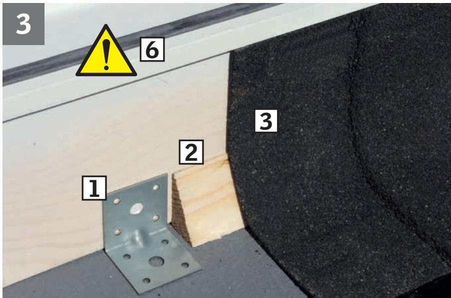
**ENGLISH:** Secure the frame to the roof construction with a minimum of two installation brackets on each side (1). Fit triangular moulding (2). Fit roofing felt on all sides (3). Cut roofing felt to fit around hinges (4), (5).
